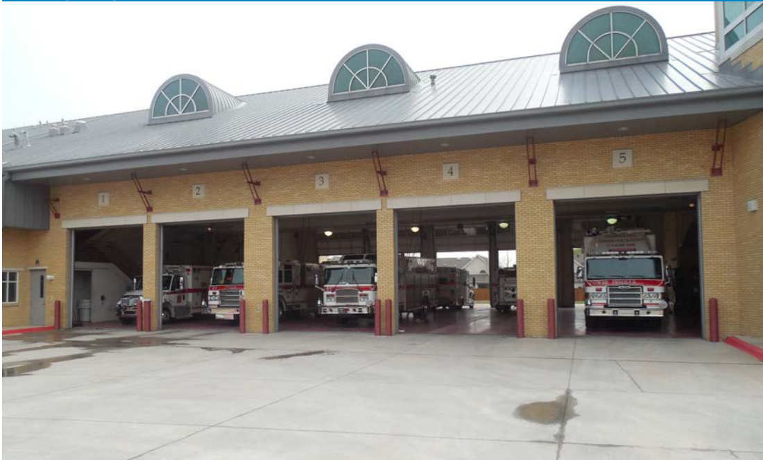
Figure 2.1 — Modern fire stations feature wide-open apparatus bays with drive-through capabilities.
