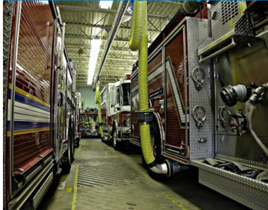
Figure 6.12 — A typical source capture exhaust filtration system.
