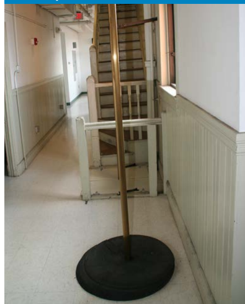
Figure 5.5 — There should be protective padding at the bottom of a slide pole.
