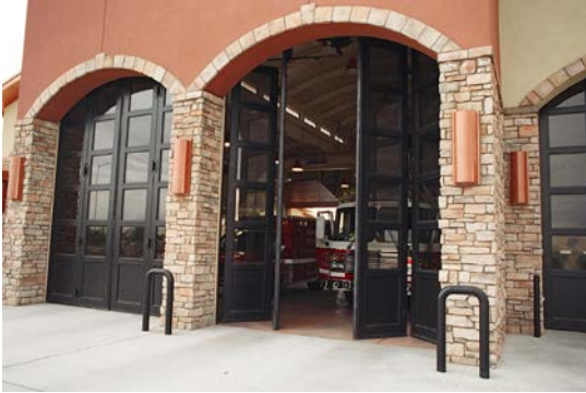
Figure 4.11 — One exterior view of a folding bay door.
