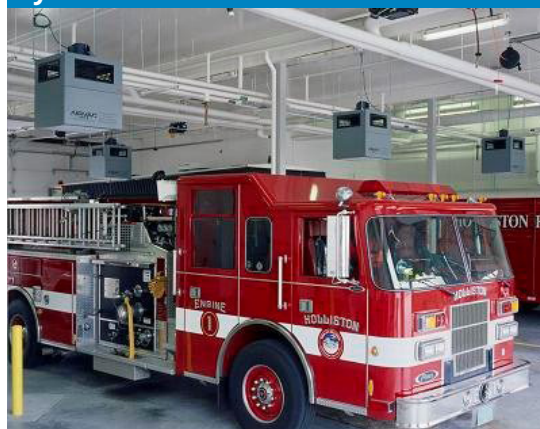
Figure 6.11 — A forced-air filtration system.
