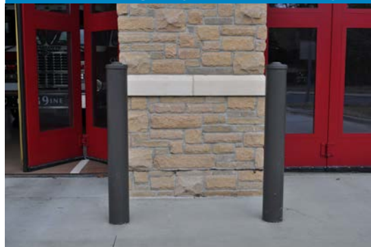
Figure 7.3 — Exterior bollards properly “inset” to protect the structure of a fire and emergency services facility.
