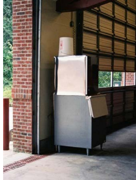
Figure 6.15 — Ice machines should not be placed in areas subject to exhaust or other contamination.
