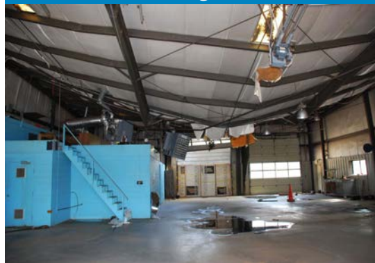
Figure 5.6 — As a result of a storm, this station roof buckled under the excessive water weight.
