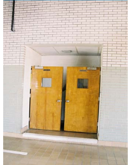
Figure 7.1 — One door leads from the kitchen and one from the dayroom; both are hinged on the wrong side. There is also a hazardous step-down to the apparatus bay.
