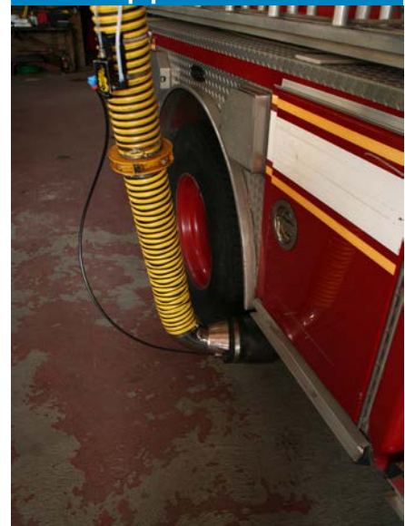
Figure 4.14 — Exhaust removal systems only work if the hose is hooked to the vehicle's exhaust pipe.
