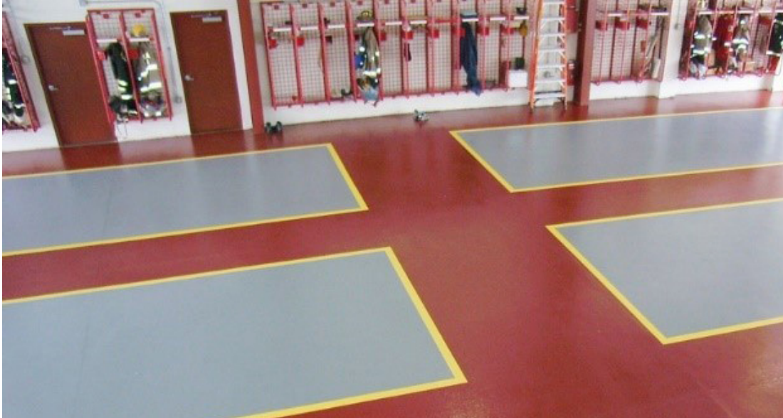
Figure 7.7 — Floor markings composed of a slip-resistant floor coating designate passageways and parking alignment.
