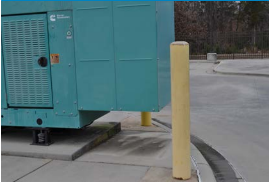
Figure 7.4a — These bollards protect the station's emergency generator.
