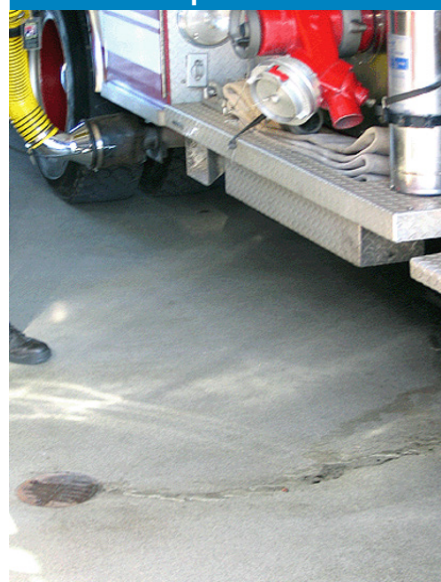
Figure 7.8 — Improper placement of apparatus floor drains create wet spots that will cause slips and falls.
